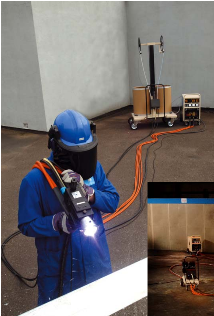
170 system spraying from drums with 10m supplies
